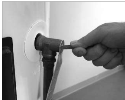
Figure 38 - T&P Relief Valve
