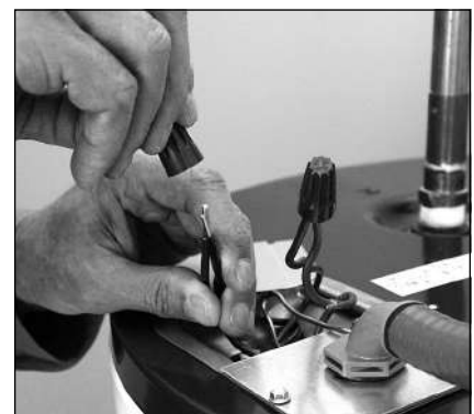
Figure 19 - Connecting the electrical wires.
