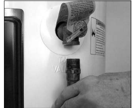
Figure 12 - Removing the T&P Relief Valve discharge pipe.
