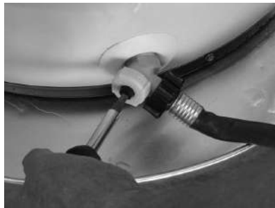
Figure 11 - Draining the old water heater.
