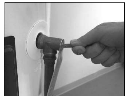
Figure 45 - T&P Relief Valve
