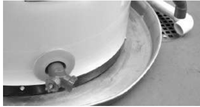
Figure 8 - A suitable drain pan piped to an adequate drain can help protect flooring from leaks and drips.
