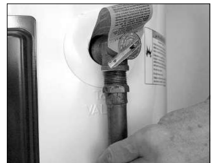
Figure 15 - The T&P Relief Valve discharge pipe must be installed properly and piped to an adequate drain.
