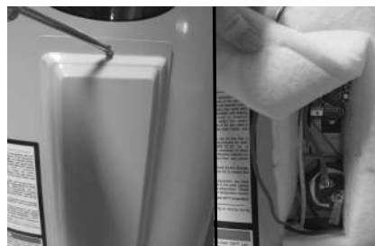
Figure 44 - Element Access Panel/ECO Compartment
