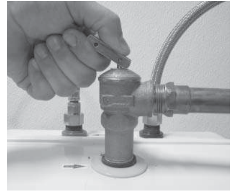
Figure 31 - T&P Relief Valve
