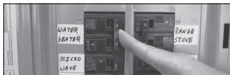
Figure 22 - Circuit Breaker
